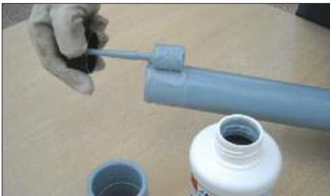
9. Apply cement to pipe and fitting. 將管配件上膠水
