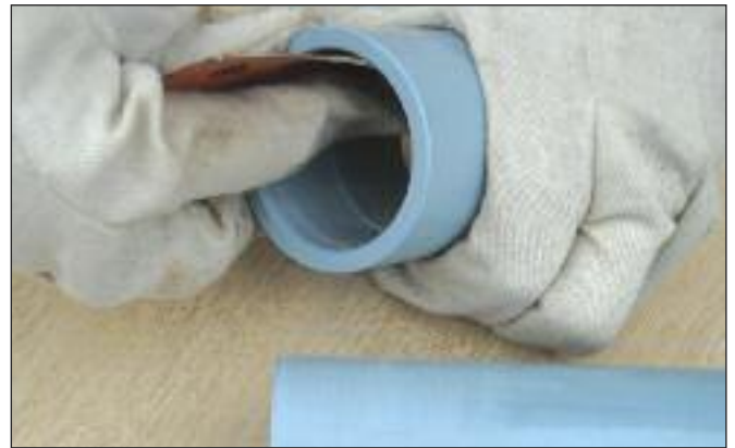
4. Abrade pipe and fitting. 摩擦管件
