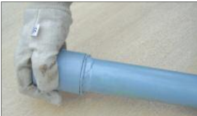
10. Push fitting home and hold for a few seconds. 將配件緊壓並停留幾秒鐘
