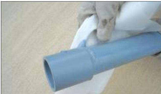
11. Cement will form a neat-bead. Wipe off excess cement with a lint-free cloth. 膠水會稍微溢出，用不起毛球布料擦拭多餘的膠水
