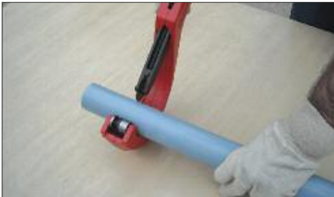
2. Cut pipe to required length. 將管件切成需要的長度
